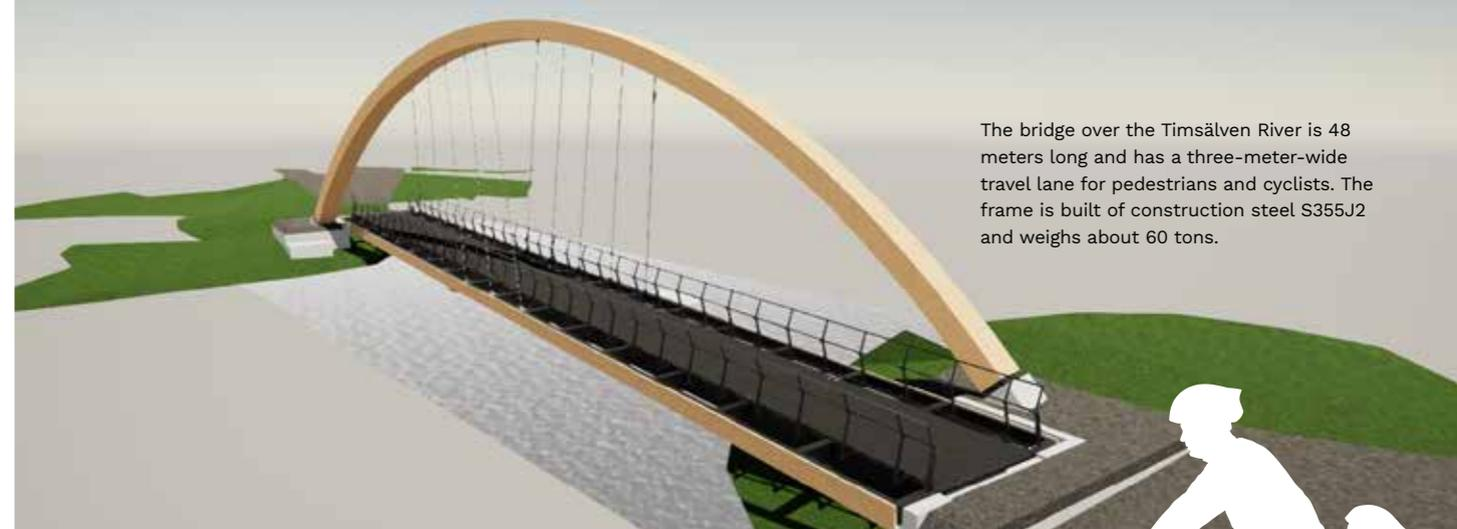
The bridge over the Timsälven River is 48 meters long and has a three-meter-wide travel lane for pedestrians and cyclists. The frame is built of construction steel S355J2 and weighs about 60 tons.
